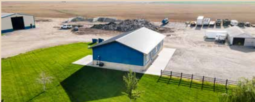
Office – Built in 2017; 60ft. x 38ft. x 12ft.
