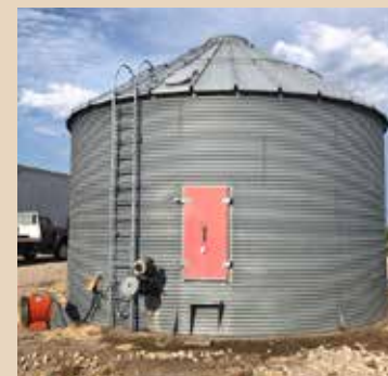
Grain Bin – 23ft. Diameter; 6,000 Bushel Capacity
